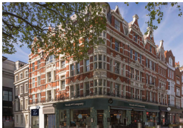
The conversion of a vacant office building on Charing Cross Road acquired for conversion by Z Hotels and co-financed by ASK and OakNorth
