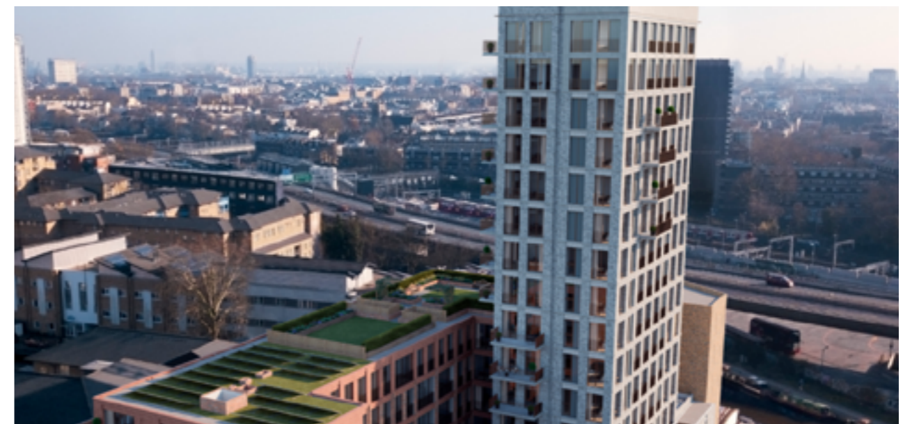
The Brick: Residential development exit loan of £25.5m provided to refinance development lender, further equity release provided after sales of 26 units
